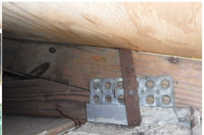
Roof to Wall Connection - single wrap straps front side
