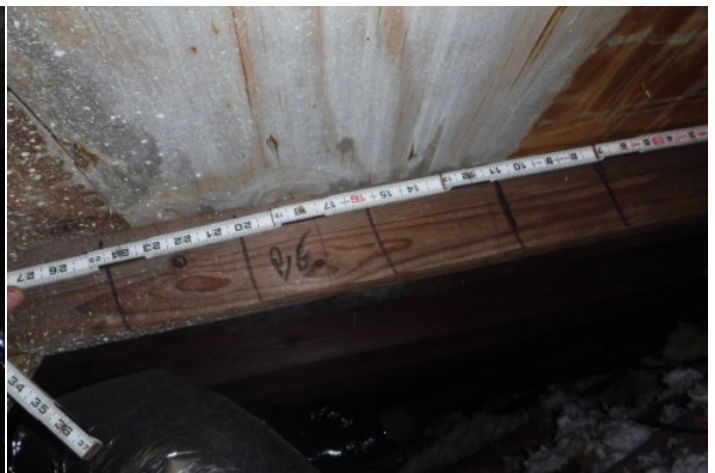
Roof Deck Attachment - 6" spacing in the field
