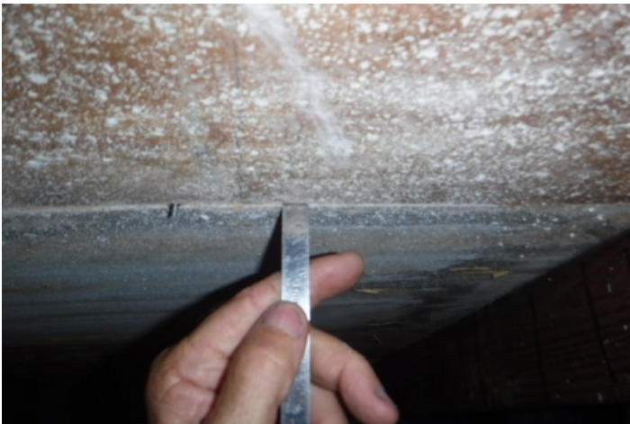
Roof Deck Attachment - 1/2" plywood sheathing
