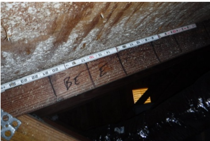
Roof Deck Attachment - 6" spacing on the edge
