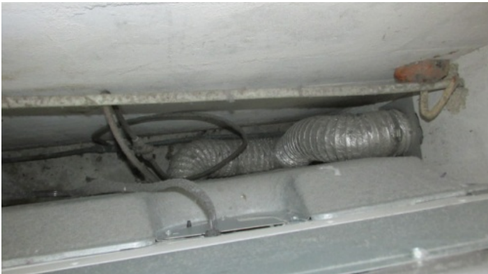
Dryer Connections
