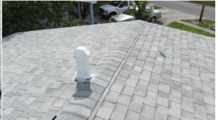
Roof penetrations looked good
