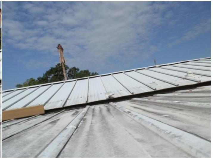
Roof Material: Metal, Rear Slope
