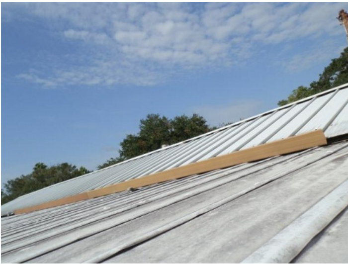
Roof Material: Metal, Rear Slope
