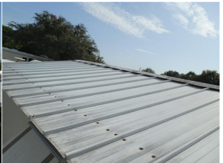
Roof Material: Metal, Front Slope
