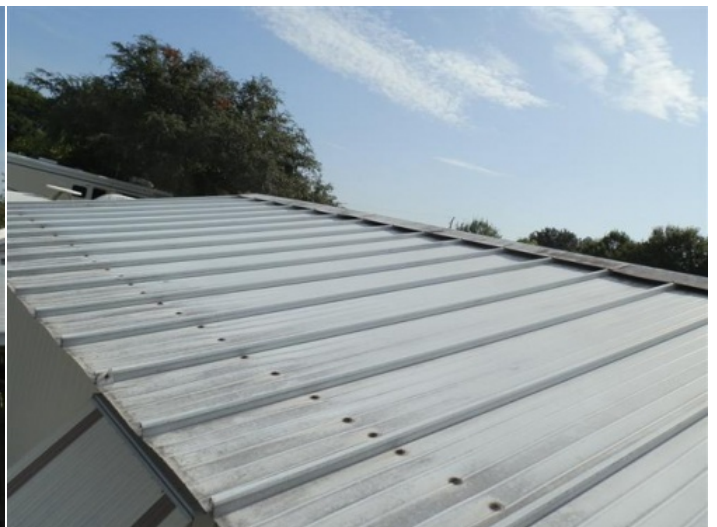
Roof Material: Metal, Front Slope
