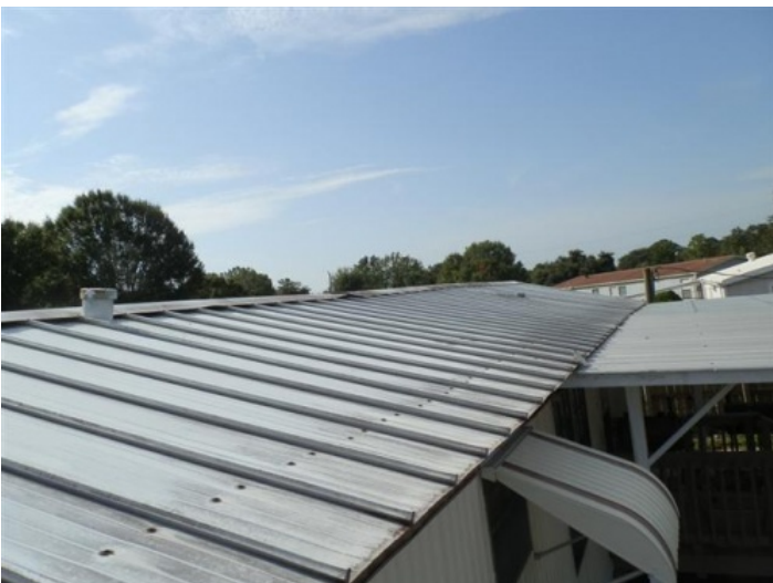
Roof Material: Metal, Front Slope
